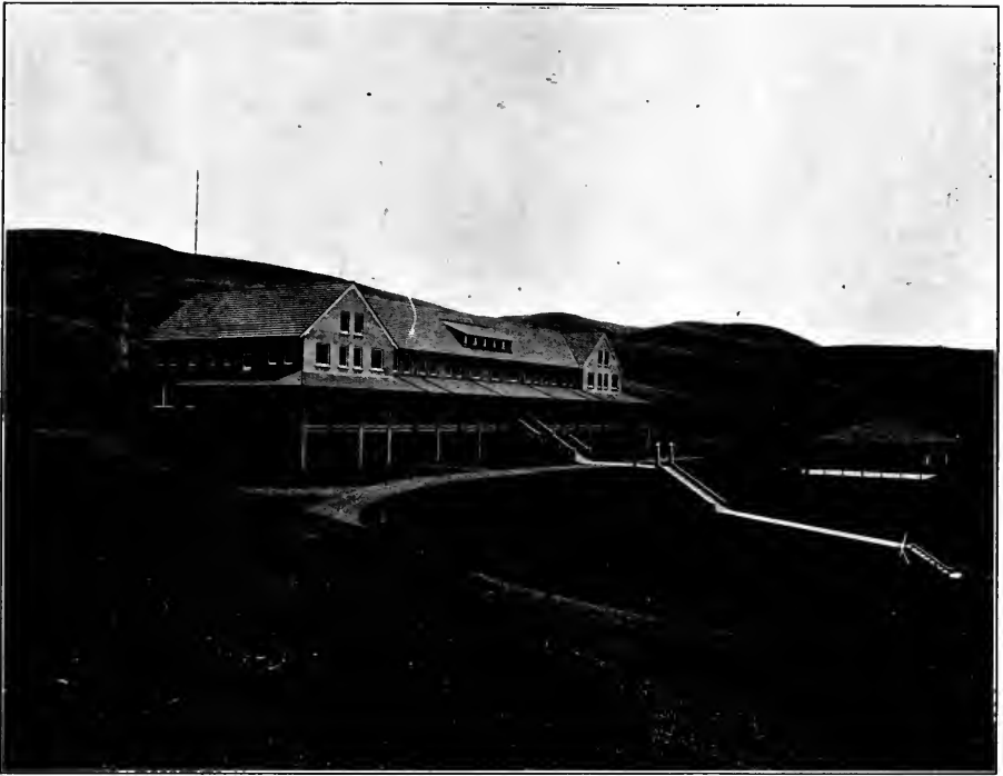
The hotel built by the Marconi Wireless Telegraph Company to house its employees at the big receiving station at Marshall, California.
